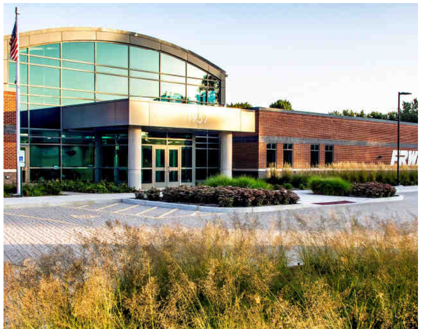
Permeable parking lot at FRWRD headquarters. Photography: DLA Architects, Ltd. / Alexander Romanovsky
