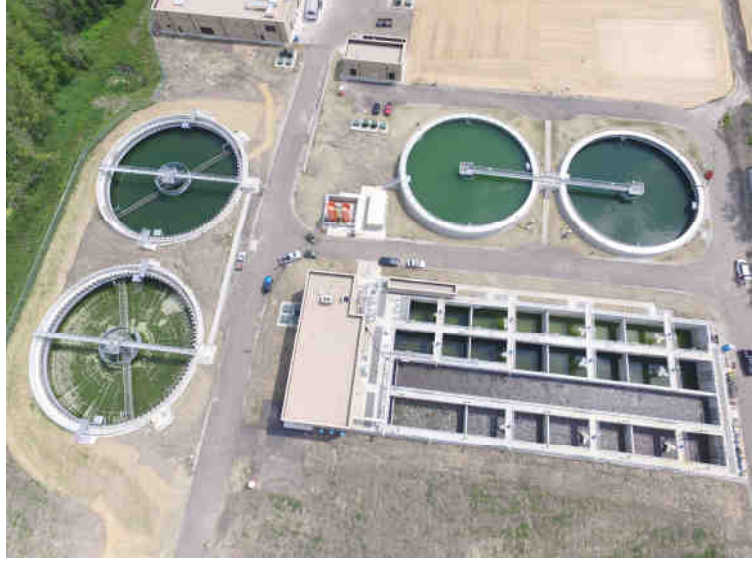
Newly Constructed Facilities for Enhanced Phosphorus Treatment at Fox Metro South Plant, Photo Credit: Fox Metro Water Reclamation District
