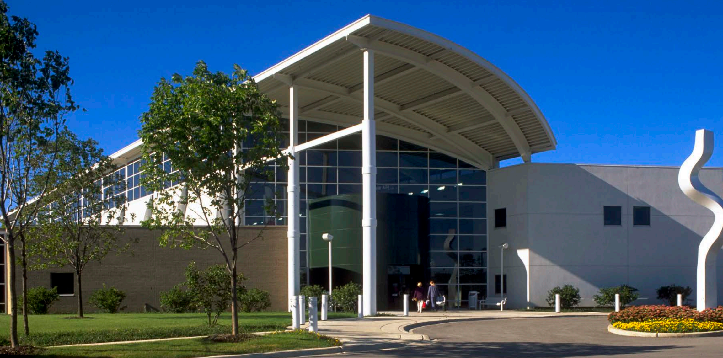
Northwest Community Hospital, Arlington Heights, Illinois
